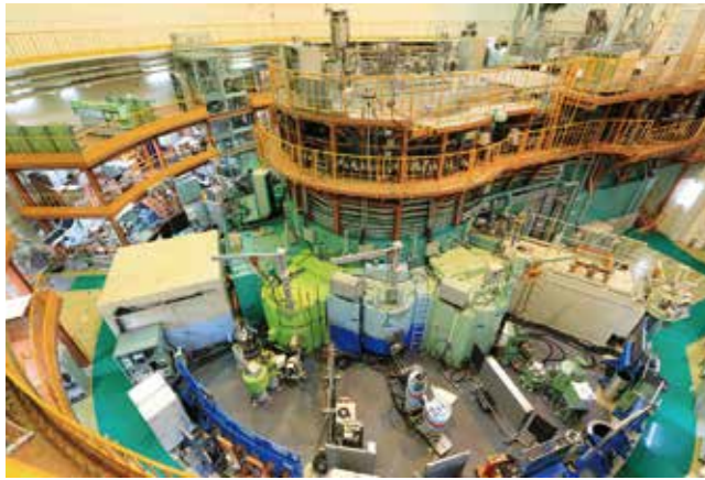
View of the reactor room
